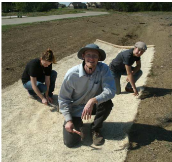
Laying down Curlex® erosion control blankets to prevent further erosion.
